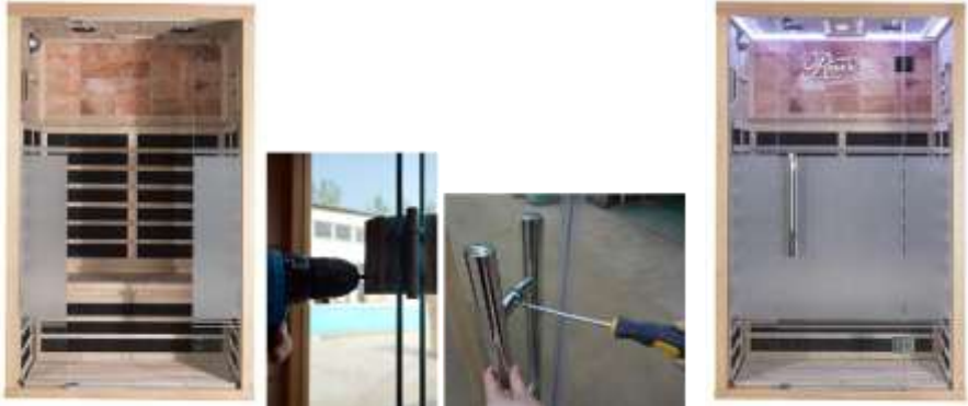
Figure I-5: Windows and Door Installation
